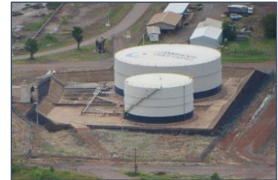
Crude storage tanks in Wyndham
