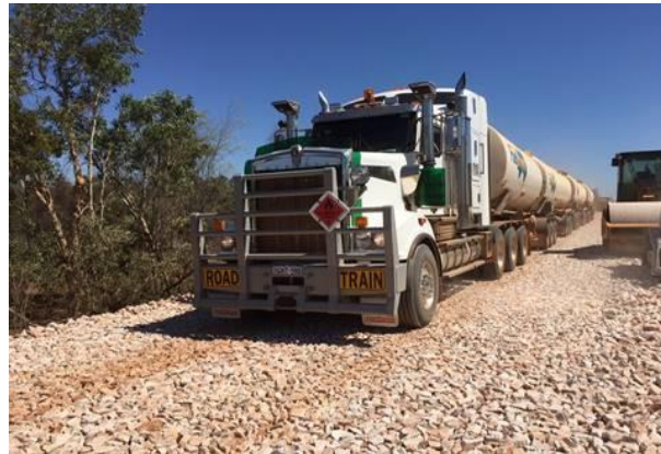
First FTA quad on Ungani access road
