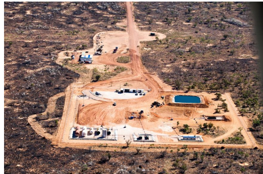
Aerial view of current Ungani Oilfield facilities
