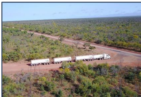
FTA quad at intersection of Ungani road and GNH
