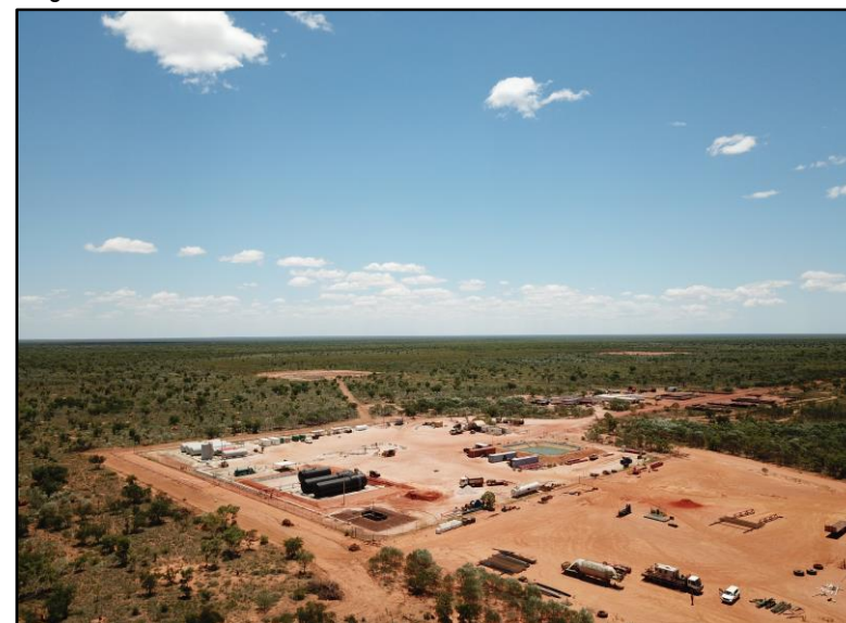
Ungani field facility
