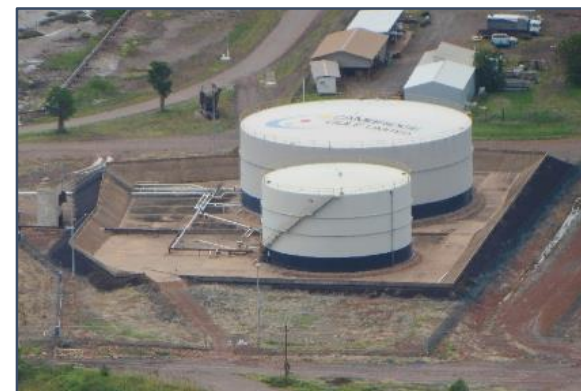
Crude storage tanks in Wyndham
