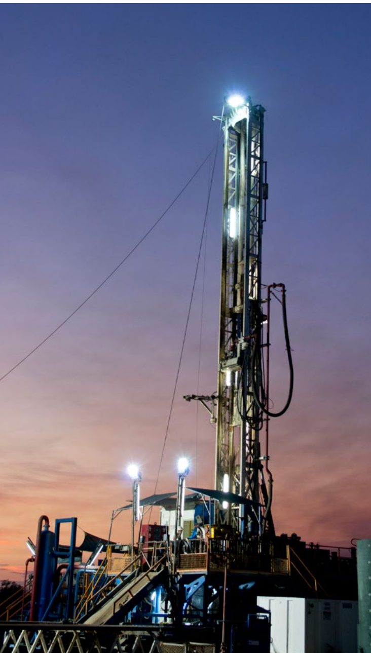
DDGT 1 drilling rig
