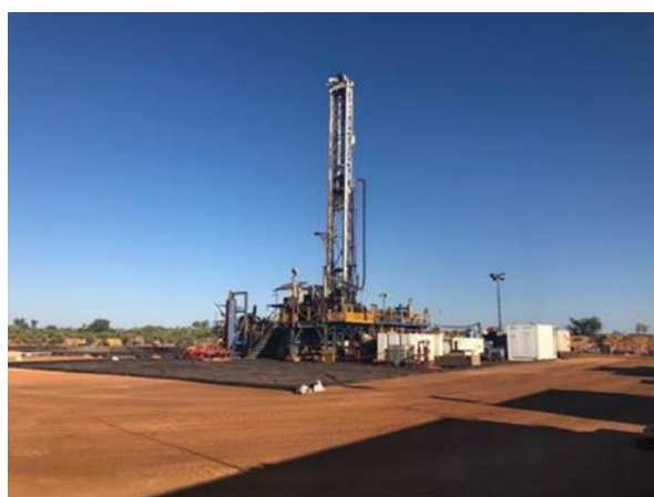
DDGT1 Rig at Ungani 4ST1
