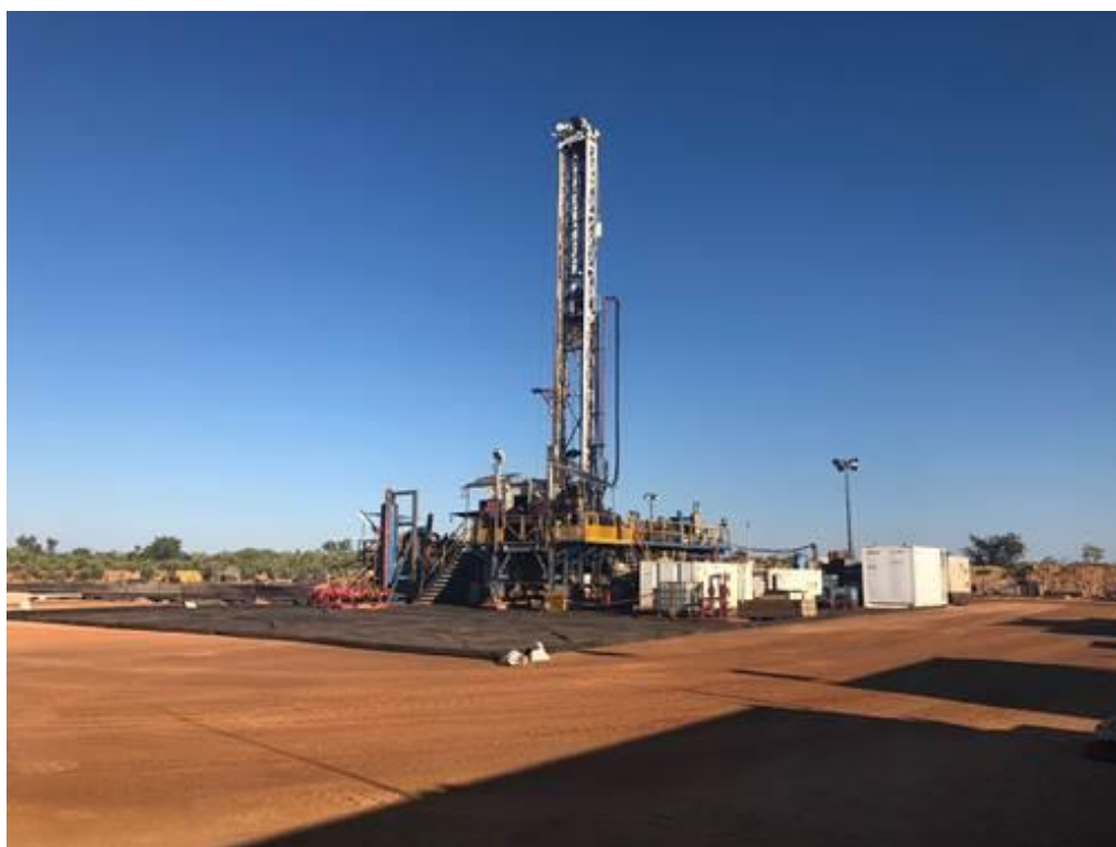
DDGT1 Rig on Ungani 4ST1 well location
