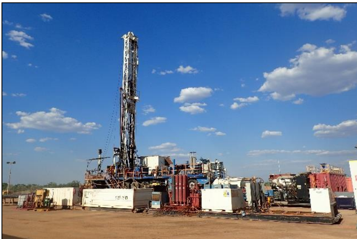
DDGT1 Rig on Ungani 4 well location
