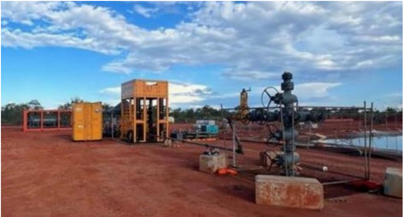
The Rafael-1 well site. Source: Buru Energy
