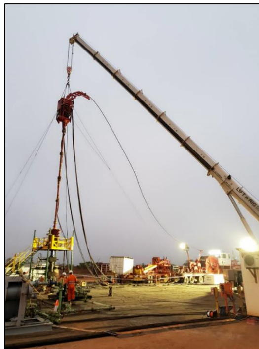
Coil tubing operations at Ungani 7H
