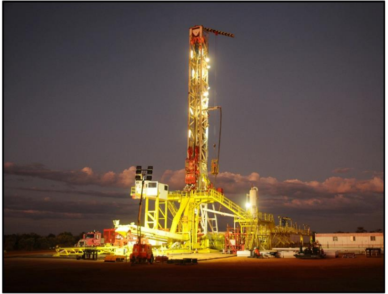
NGD 405 drilling rig
