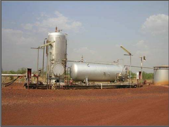
Blina oilfield facility
