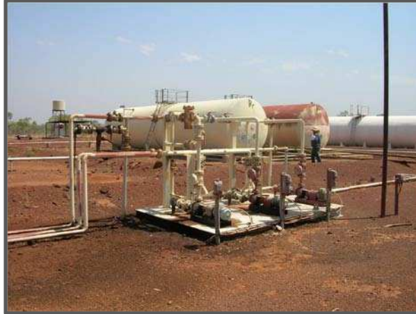
Meda load-out facility
