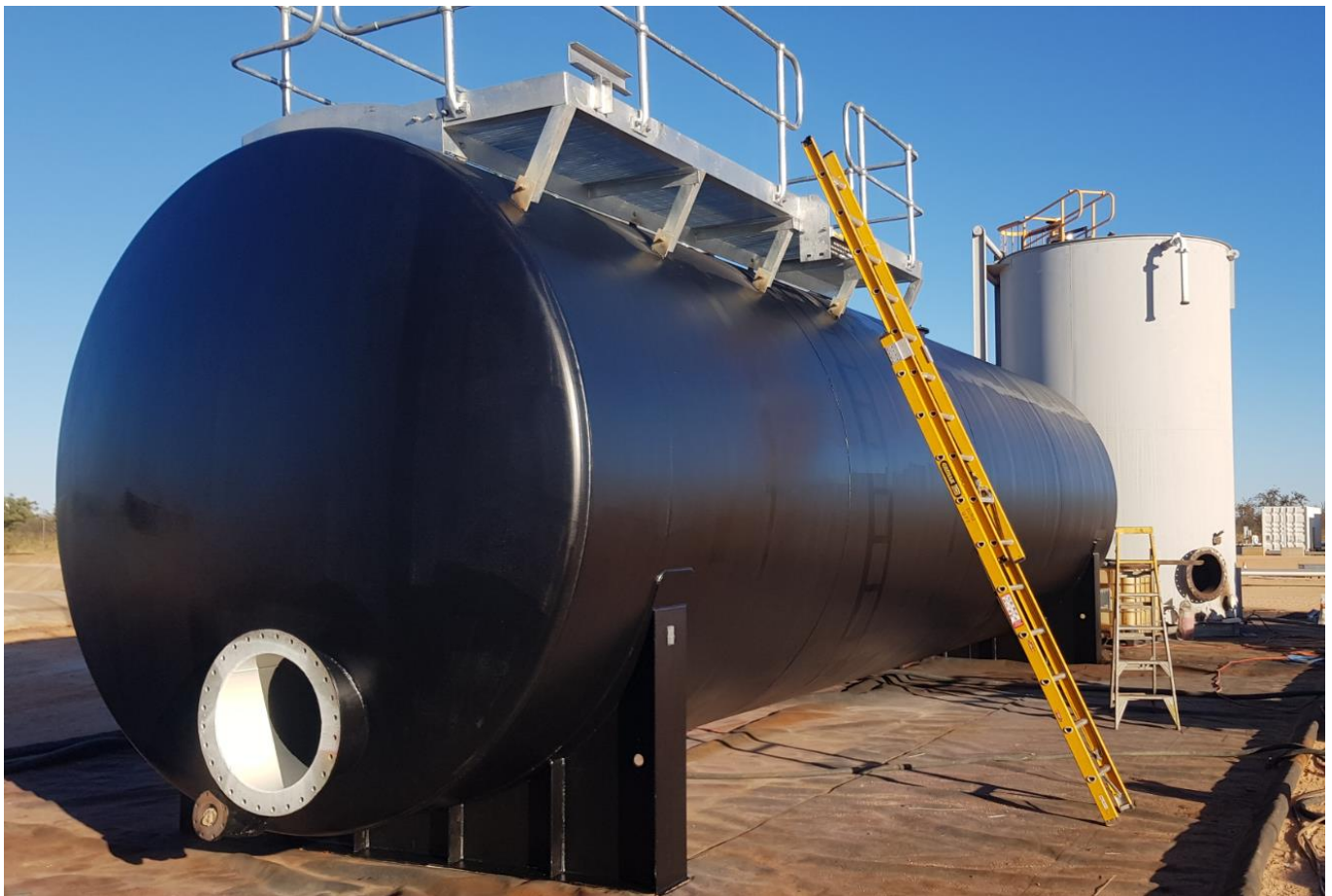
Installation of additional fluid separation tanks at the Ungani Production Facility
