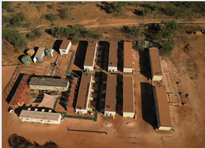
Buru jacking platform workover crew and Ungani camp
