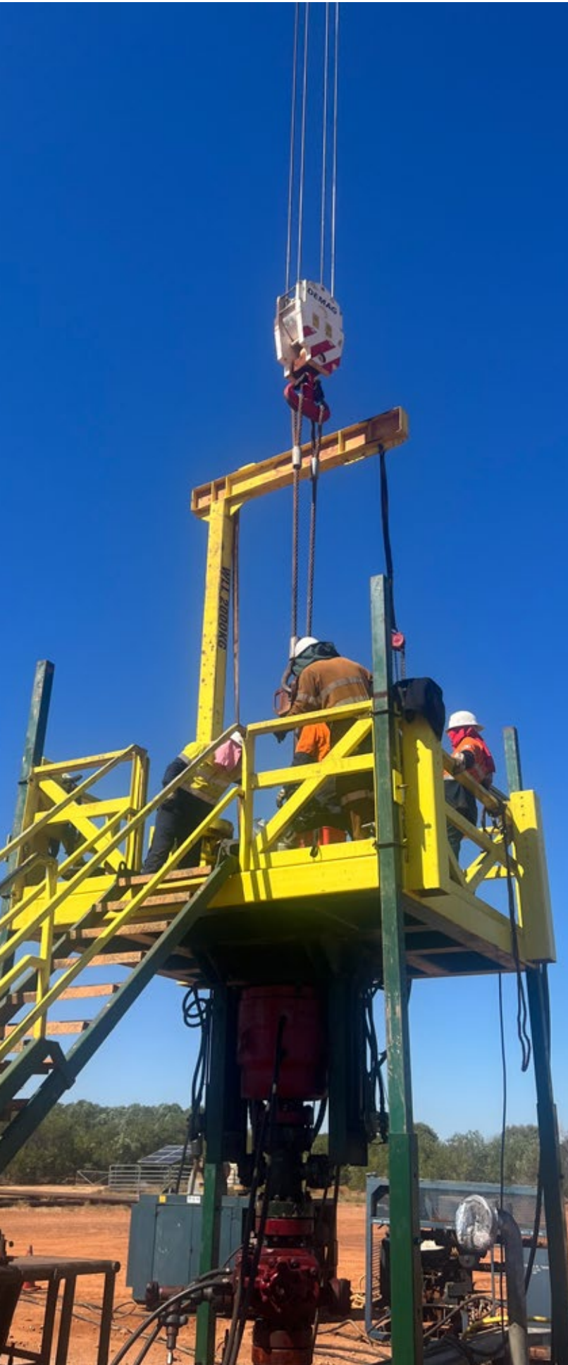
Ungani 5 well maintenance with Buru jacking platform system
