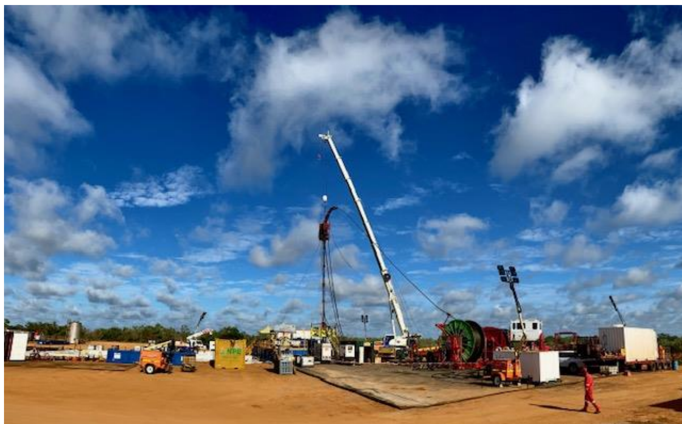
Coil tubing operations on the Ungani 6 well
