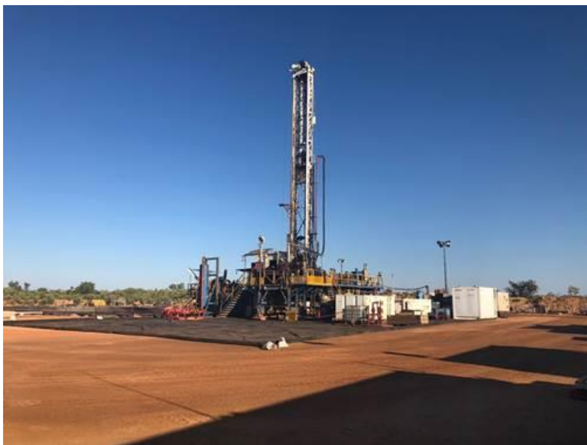
DDGT1 Rig on Ungani 4ST1 well location
