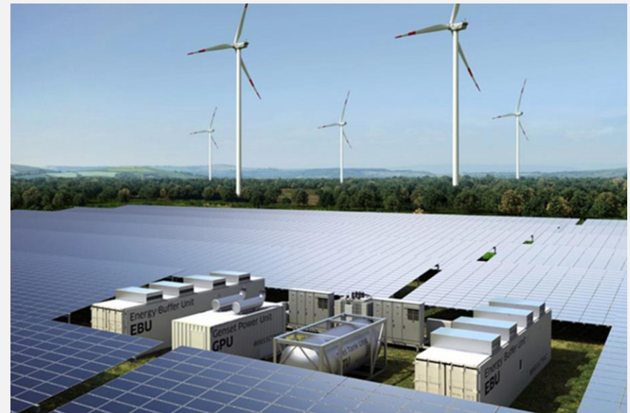
Source: Grid-integrated hybrid technology (belectric.com)
