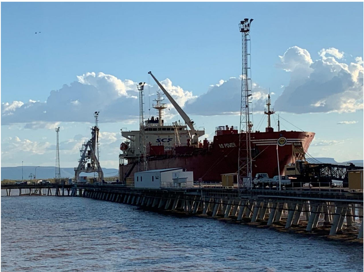
Ungani crude lifting at Wyndham in November by the NS Power
