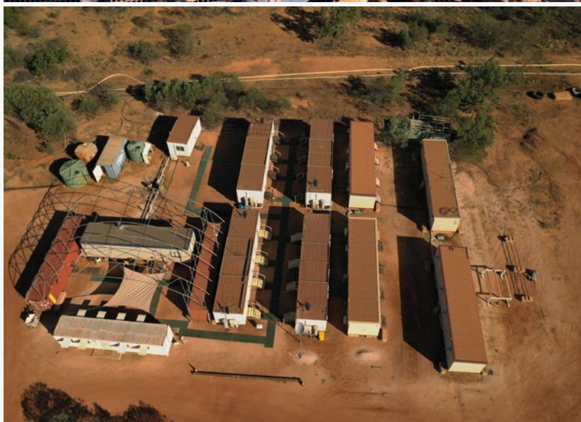
Buru jacking platform workover crew and Ungani camp
