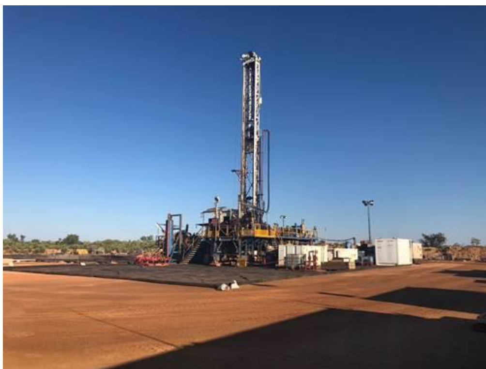
DDGT1 Rig on Ungani 4ST1 well location
