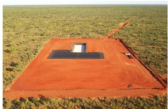
Rafael 1 drill pad ready for rig location
