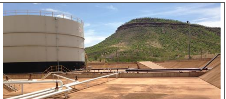
Wyndham Tank Farm and Piping Modifications
