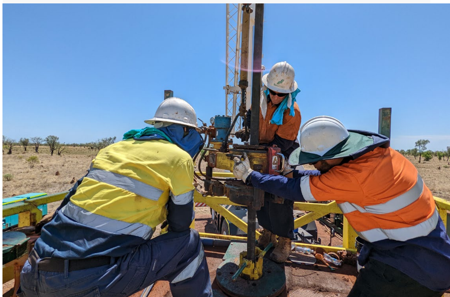
Well decommissioning operations
