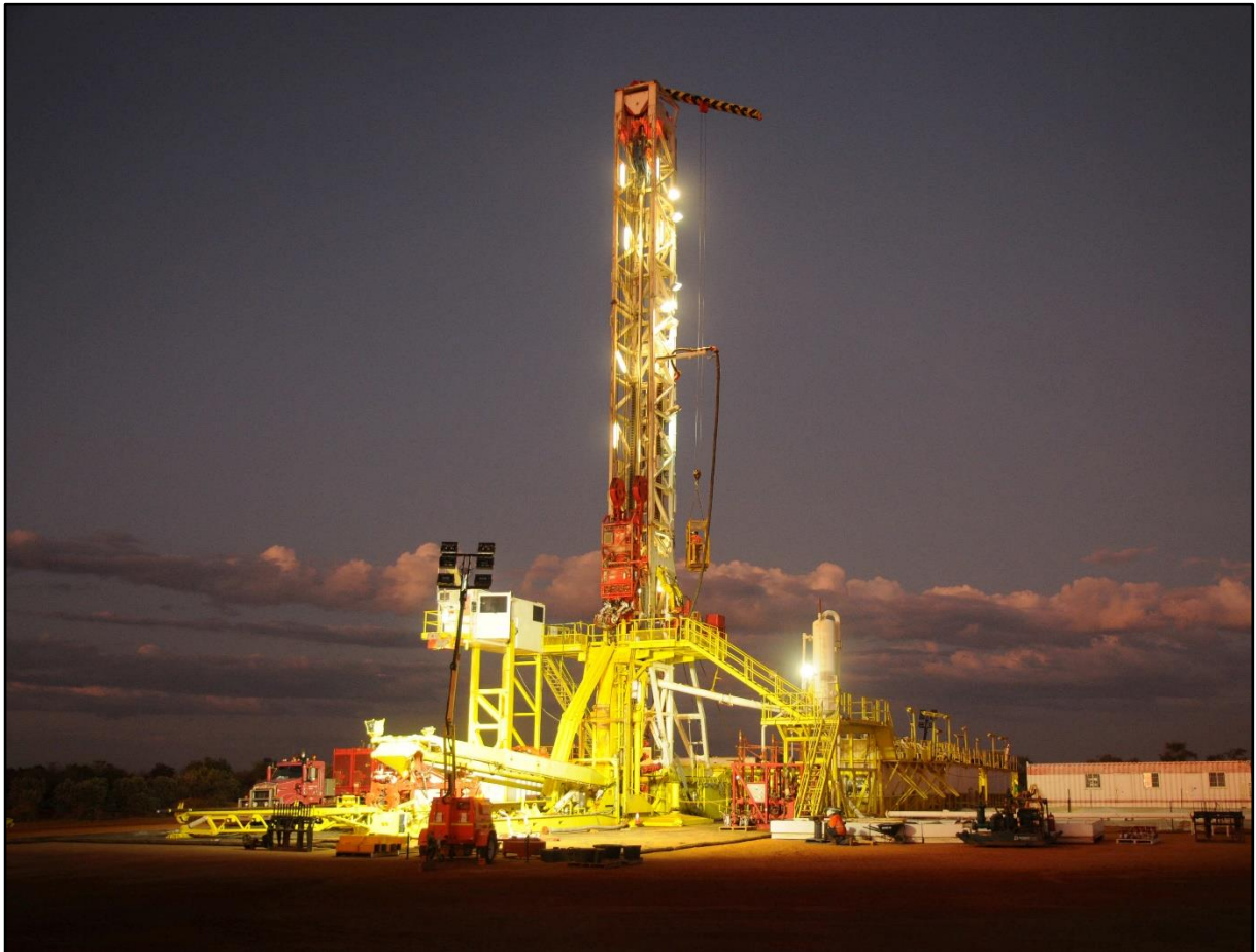
NGD 405 rig at Ungani 6 location
