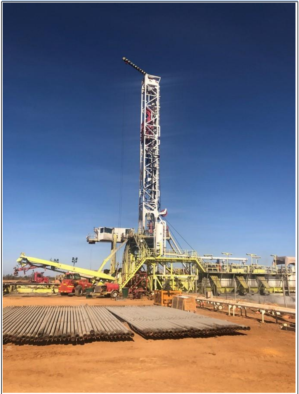
Fig. 1: BRU's Jacking Platform
