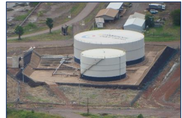
Wyndham Tank 10 (at rear)
