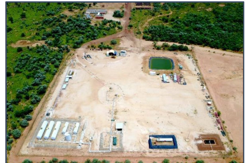
Ungani field facility
