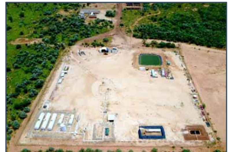
Ungani field facility
