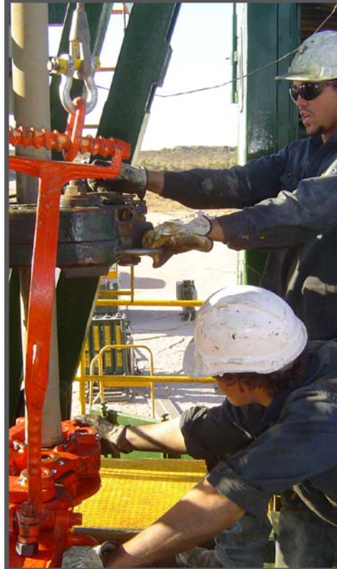
Drilling operations on the Fairway Rig
