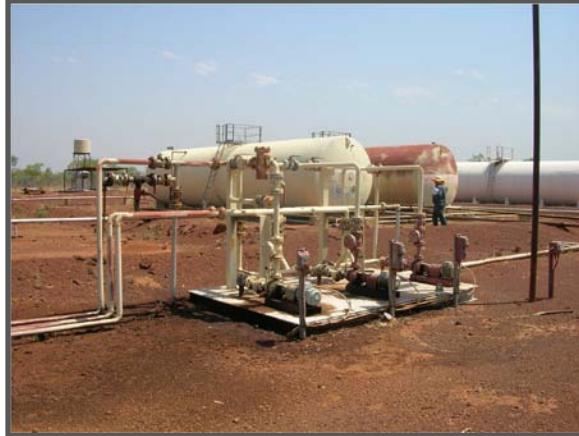
Meda load-out facility
