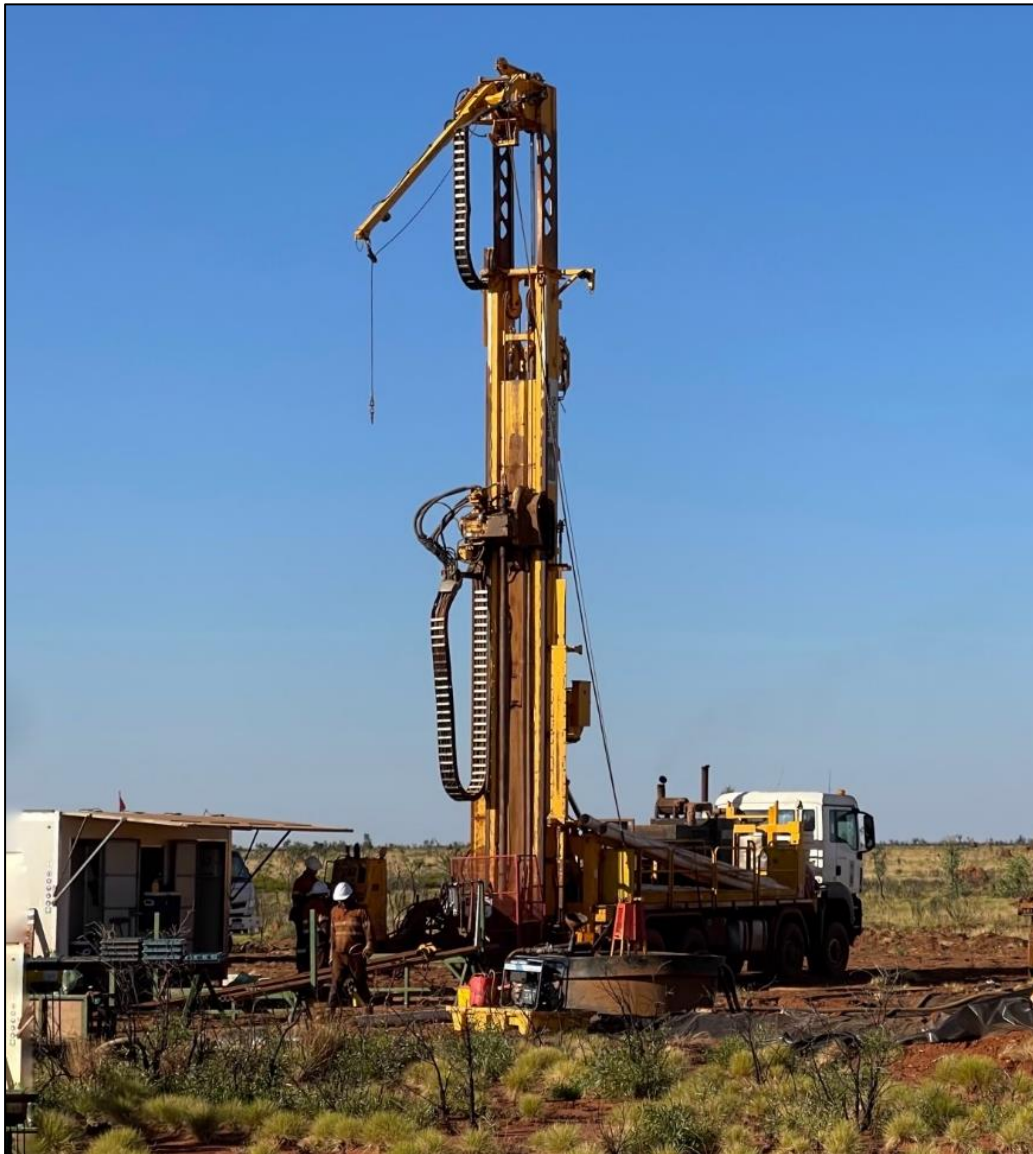
Figure 1: Diamond drill rig commencing drilling at the Barbwire Terrace project.
