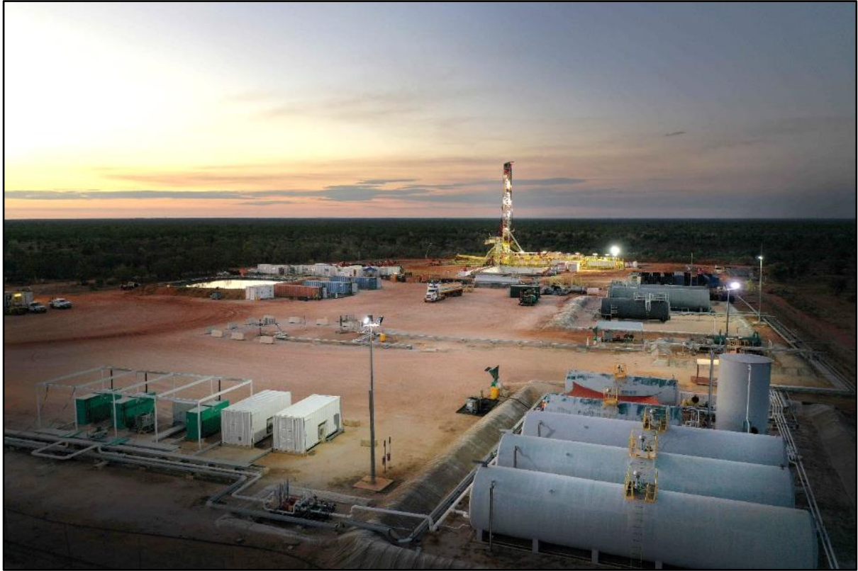
Ungani Production Facility and NGD 405 rig at Ungani 6 location
