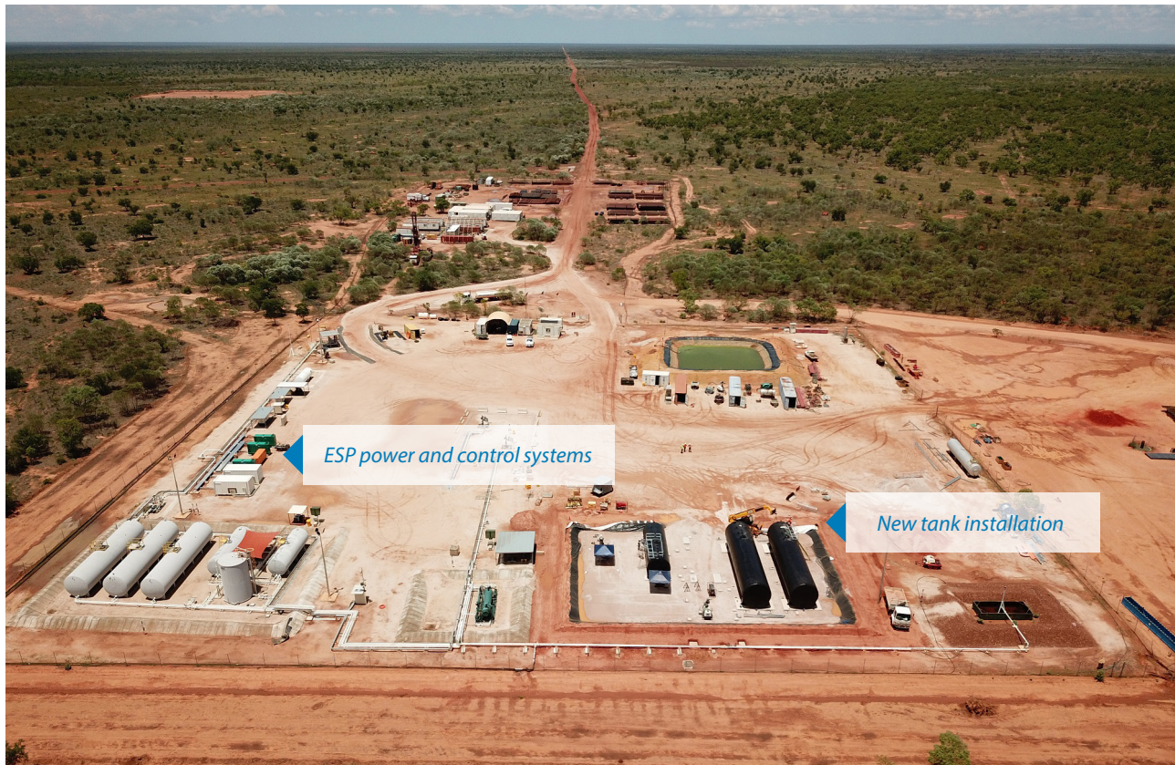
Ungani Production Facility showing ESP surface equipment and new tank installation
