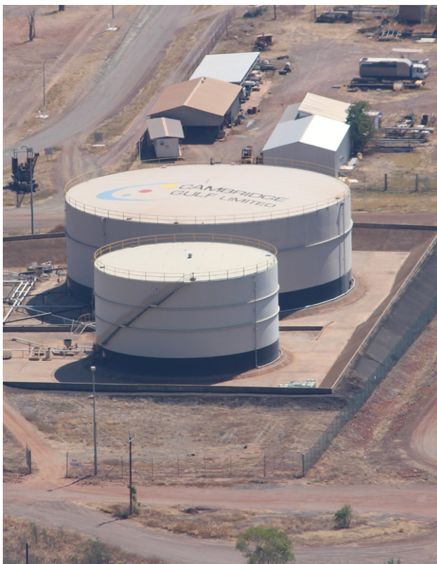
80,000 bbl and 30,000 bbl tanks at Wyndham
