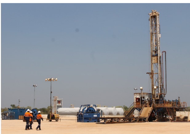
DDGT1 Workover Operations at the Ungani 1ST1 well
