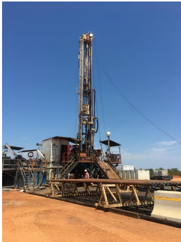
DDGT1 Rig on Ungani 5 well location
