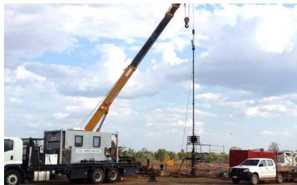
Ungani North 1 well testing operations
