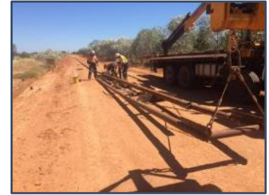
New flowline being laid
