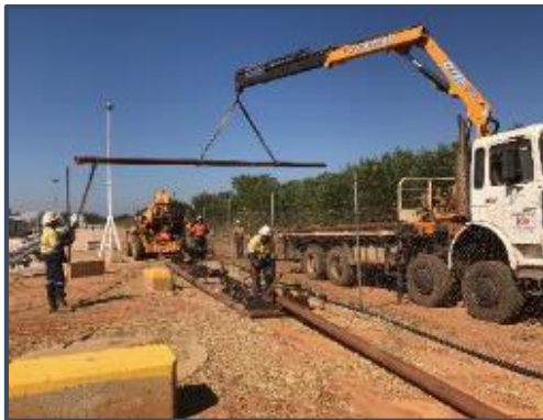
Flowline works at Ungani production facility
