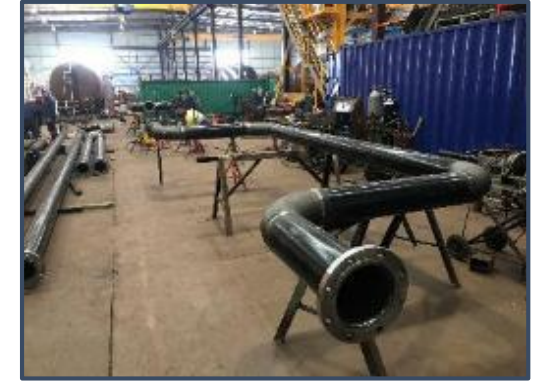
New tank piping fabrication
