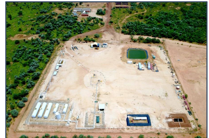
Ungani field facility
