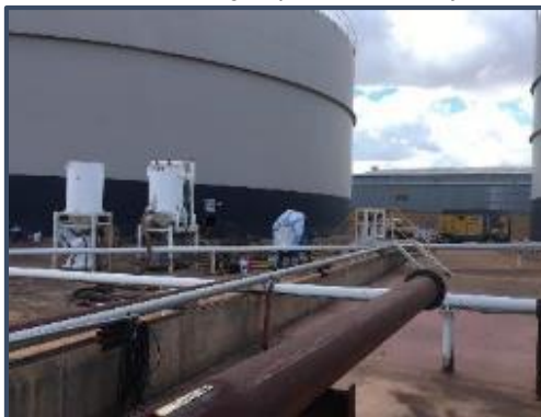
Tank preparation works at Wyndham
