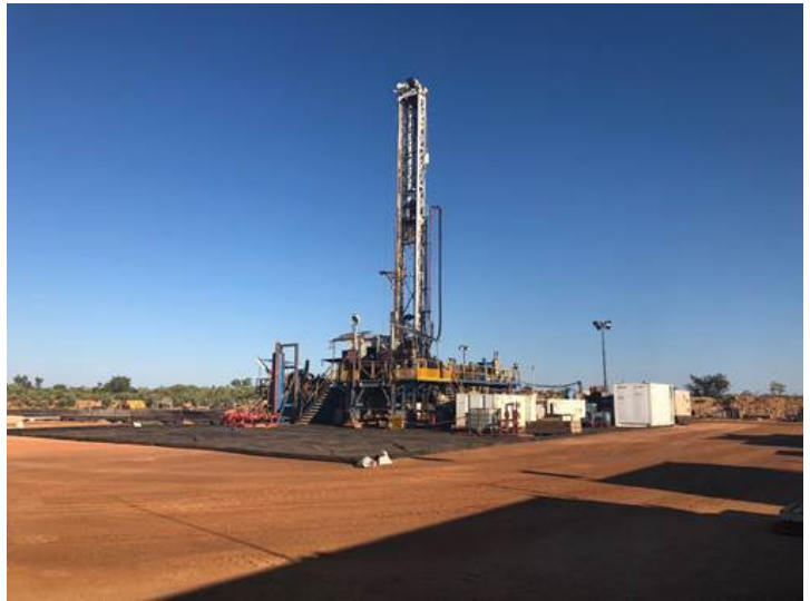
DDGT1 Rig on Ungani 4ST1 well location
