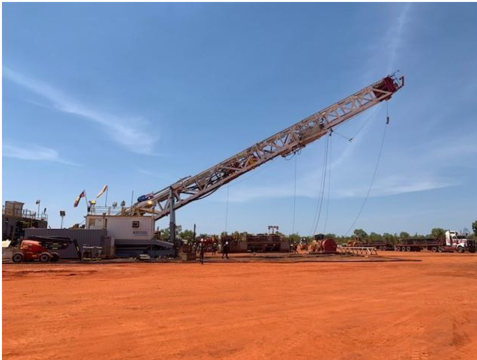
Ensign 963 mast lowering for move to Ungani 8
