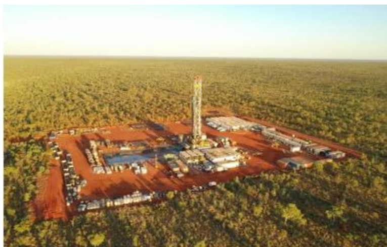
Figure 9: Rafael well site during drilling.
