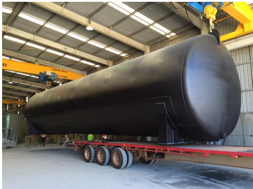
1,250 bbl storage tank under construction
