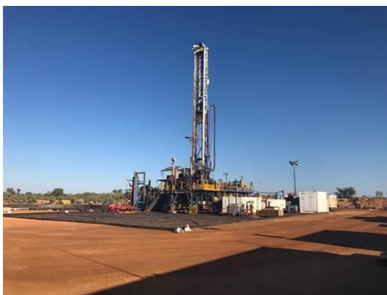
DDGT1 Rig on Ungani 4ST1 well location
