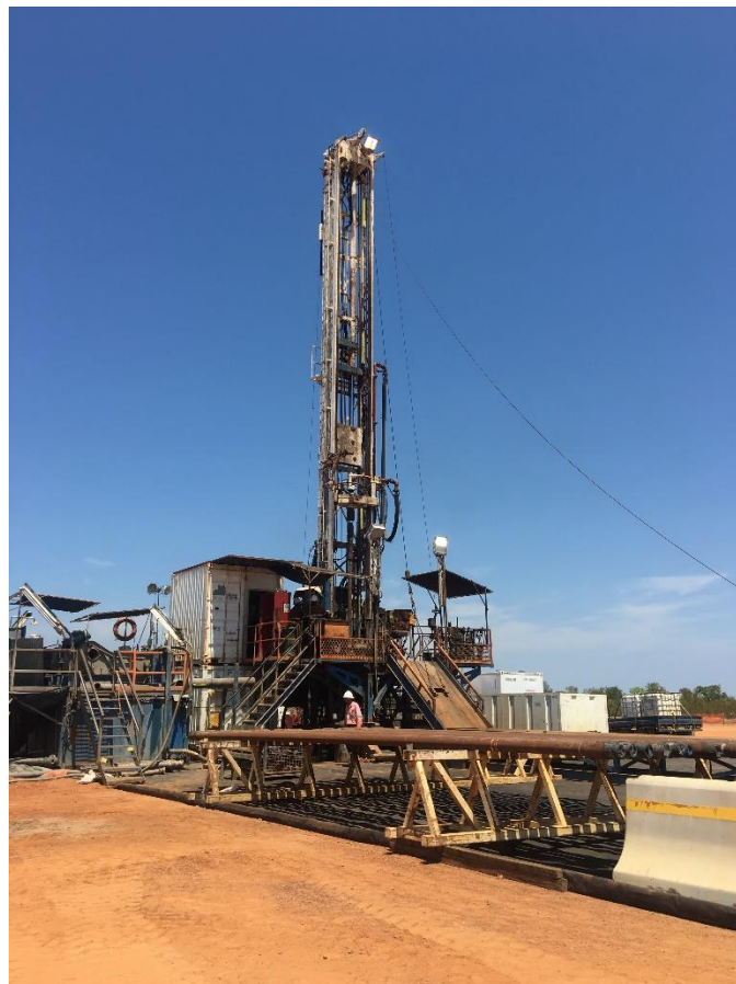
DDGT1 Rig on Ungani 5 well location
